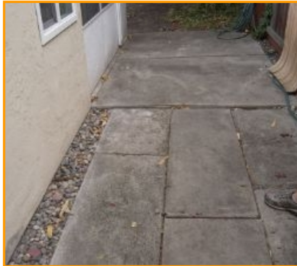
Walkway has normal wear and tear.
